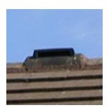
An Open Flued Appliance using a Ridge-tile flue terminal (pre1996)
