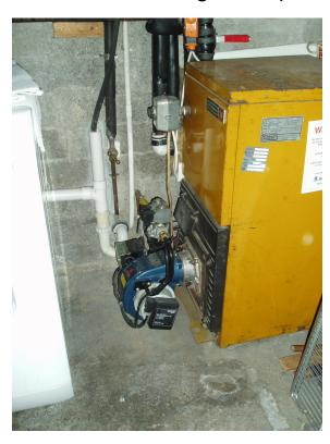
An Open Flued Boiler originally burning oil that which was converted with a forced draught gas burner for use with Natural Gas i.e. a burner to burner changeover
