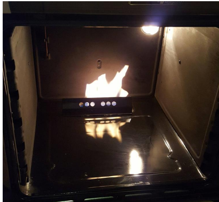
Photo 2. Bad Flame picture in oven (Nat Gas set-up with LPG in use)
