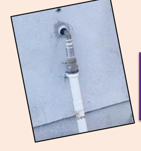
This example ticks all the boxes for gas pipework sleeving through a load bearing wall.
