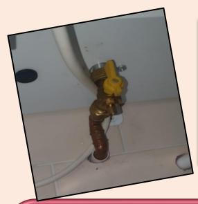
This is a common scenario where a gas supply from underneath the boiler runs through a tiled wall. The 15mm copper pipe is going through a 22mm sleeve which is too small in diameter. According to table 1, 15mm copper requires a 25mm sleeve at the minimum.
