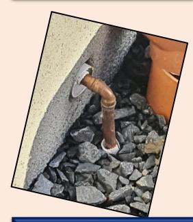
On this particular installation, whilst there is adequately sized sleeving present, the space between the sleeve and the wall was not cemented and sealed. The copper pipe was also left exposed which makes it susceptible to mechanical damage.
