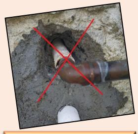
In this example, the factory coating on the copper was used as a sleeve and this is not deemed to be a suitable sleeve. The wall was also not finished correctly.
